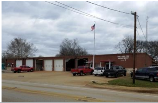
Figure 120: Bullard VFD, Station 1
